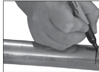
Figure 3 — Marking for Insertion Depth
