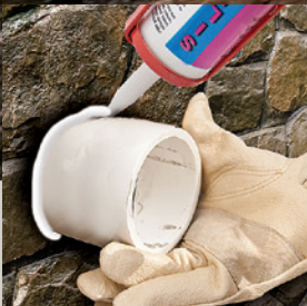
Seal wall opening with 100% silicone caulk.
