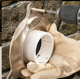
Install anti-theft escutcheon. Secure with appropriate anchor.
