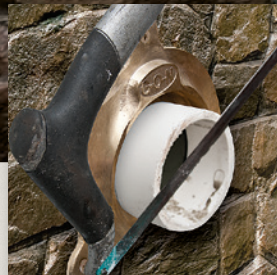
Measure hub depth of G-O-N. Cut to proper length.
