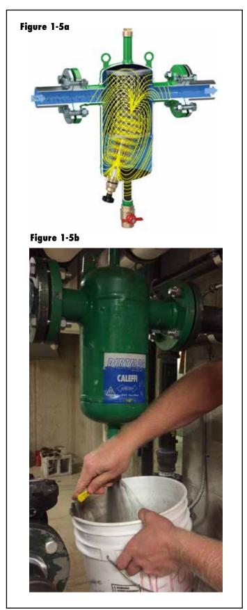
such as air and dirt removal. Devices such as microbubble air separators and magnetic dirt separators have found increasing application in North American systems. These devices have improved the performance of hydronic heating and cooling systems, and lengthened their service lives. Figure 1-5 shows an example of a magnetic dirt separator being "blown down" to remove the ferrous oxide sludge captured from within an older hydronic system.
