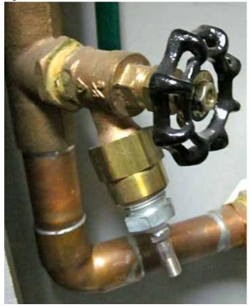
With exception of specifications that require certain test pressures, there is no universally accepted pressure to which all hydronic systems should be tested. A suggested test pressure is 1.5 times the pressure relief valve rating, *assuming that all components in the piping system have*
